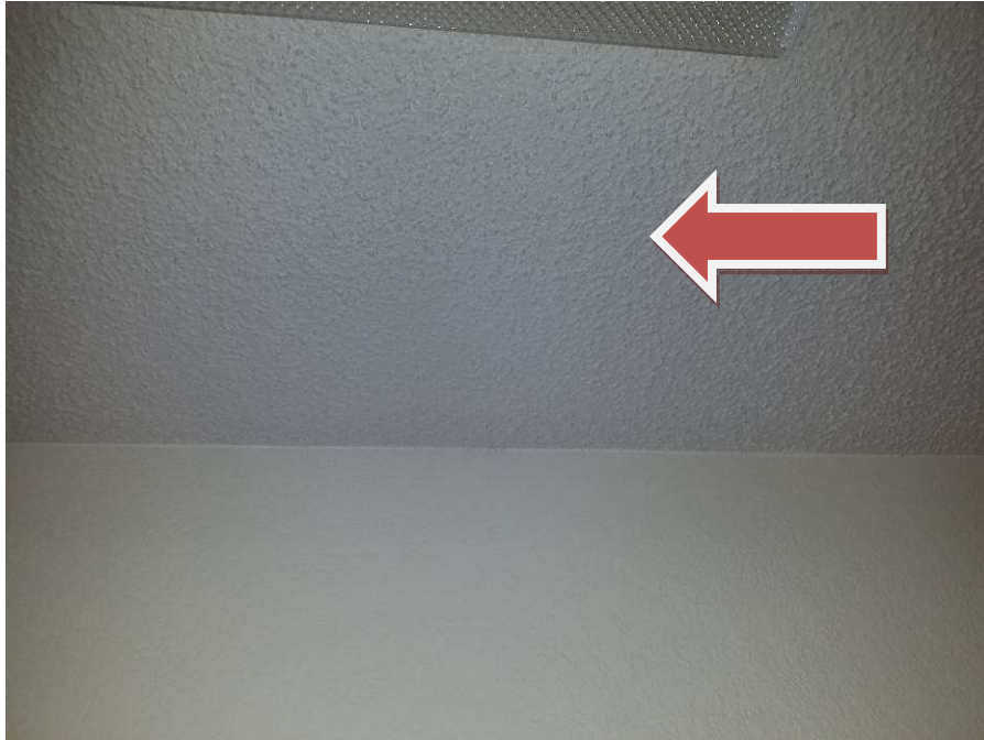
Photo 3: Typical RACM white plaster ceiling finish (popcorn ceiling) on floor 1.
