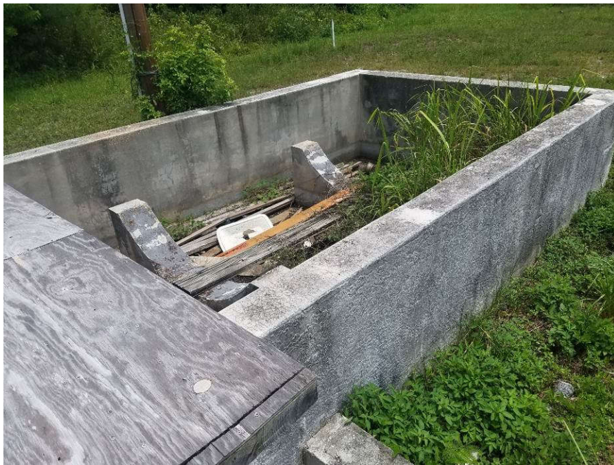
Photo 8: Concrete storage tank barrier/wall.
