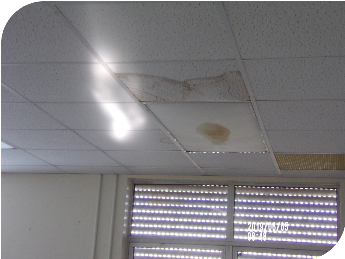
Ceiling showing evidence of leaking
