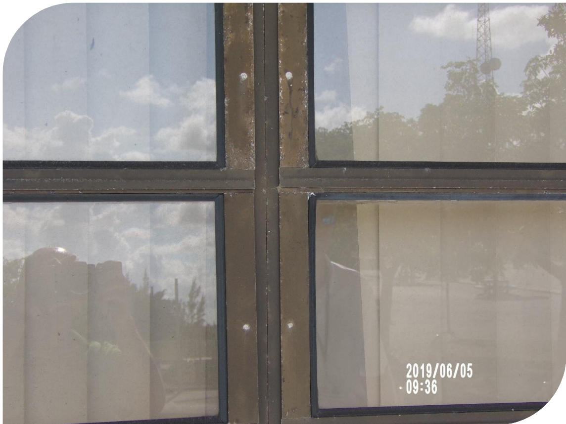
Non-rated windows with gaps that allow air intrusion
