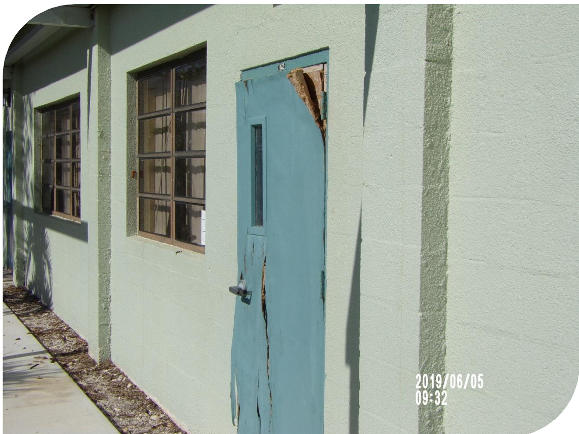
Deteriorated wood doors
