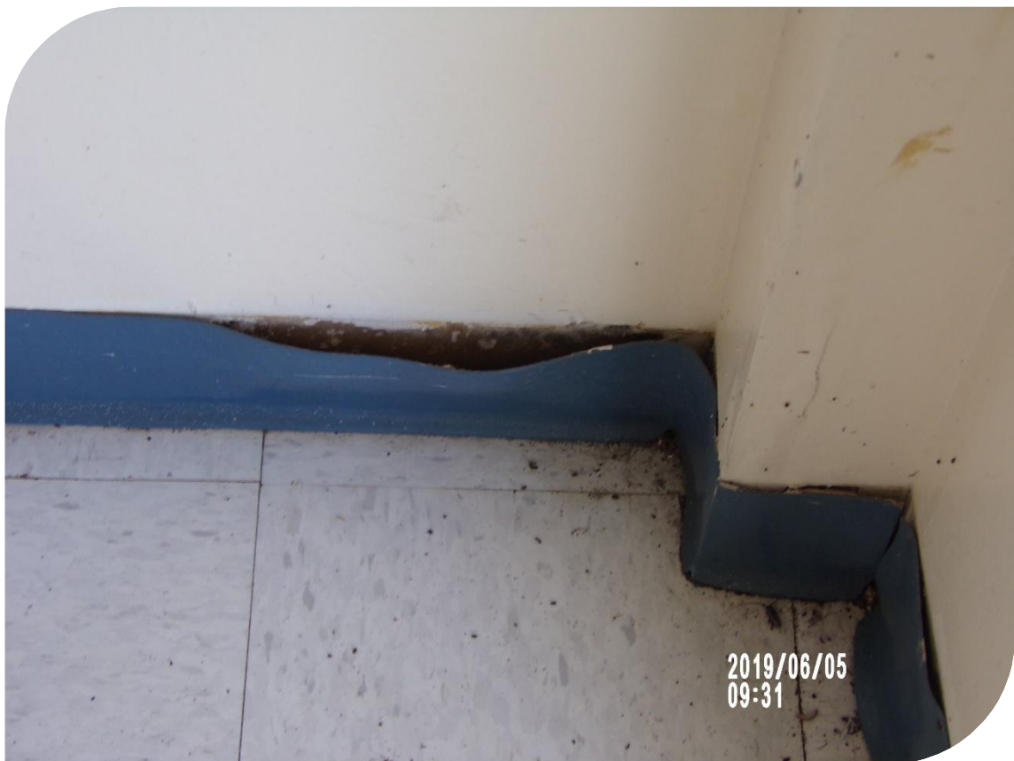
Moisture intrusion at base
