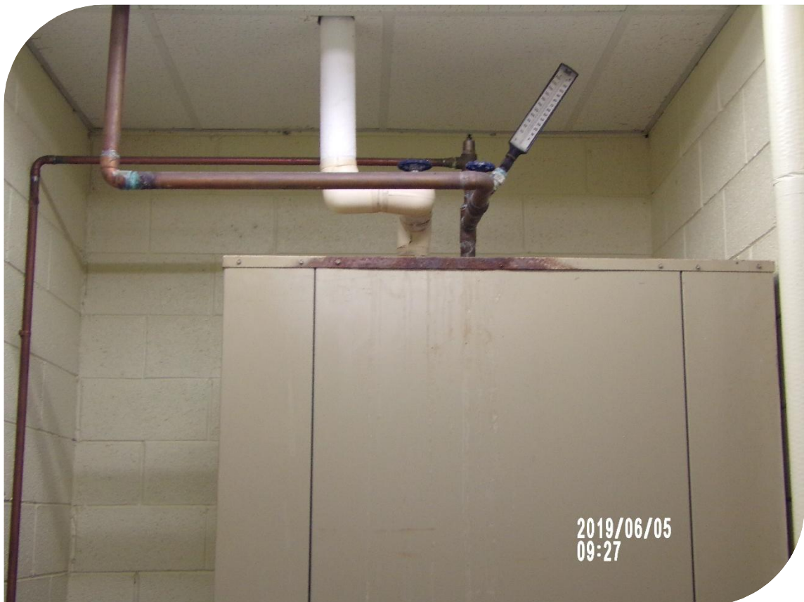
Moisture through roof damaging equipment
