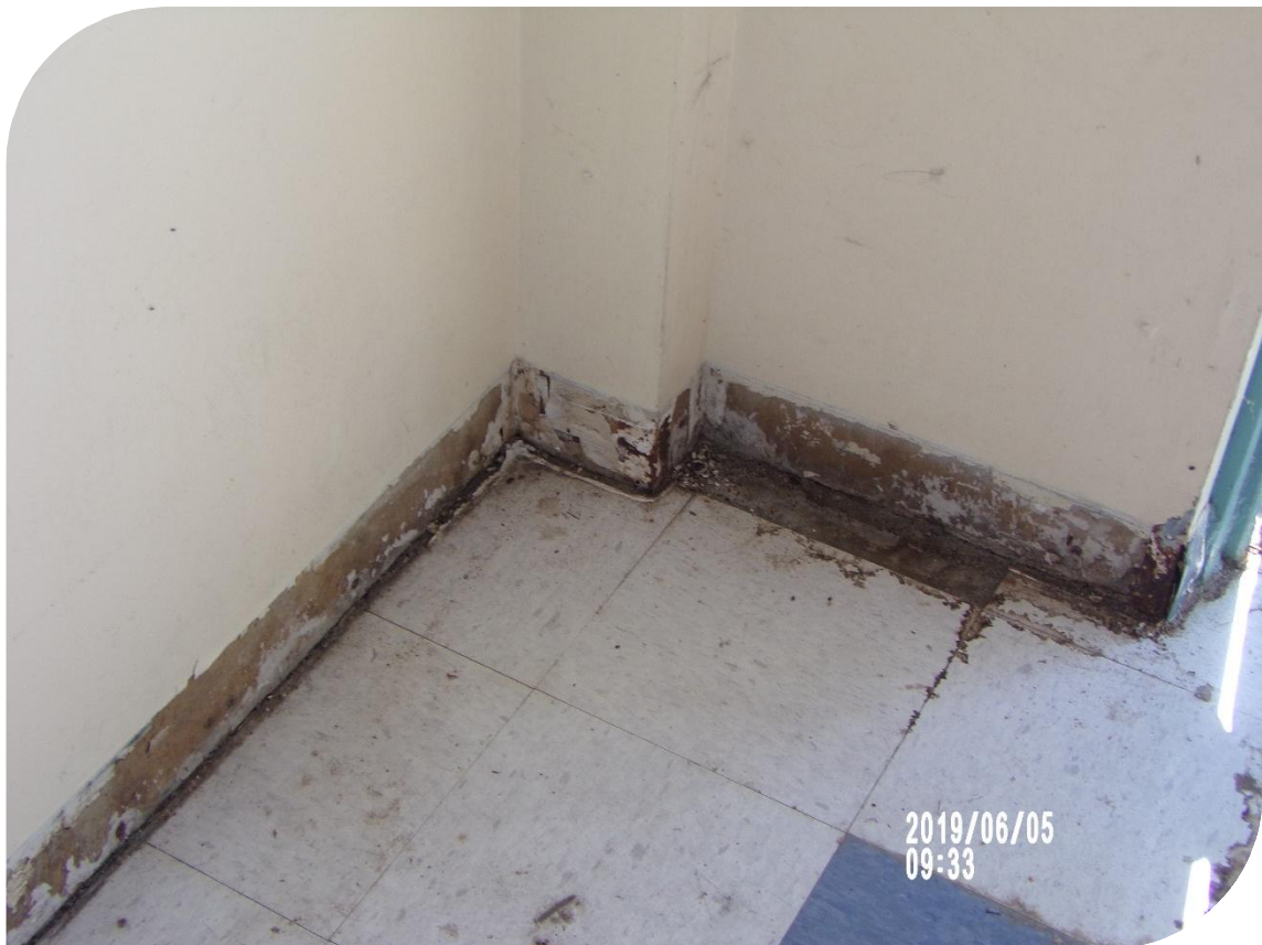
Moisture intrusion at base
