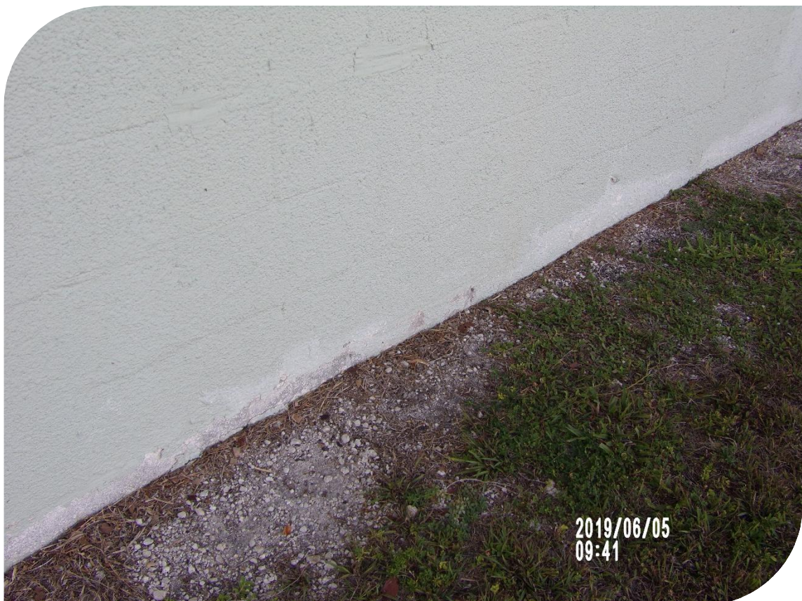
Ground around foundation washed away
