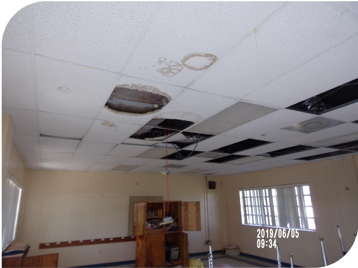
Evidence of leaking roof
