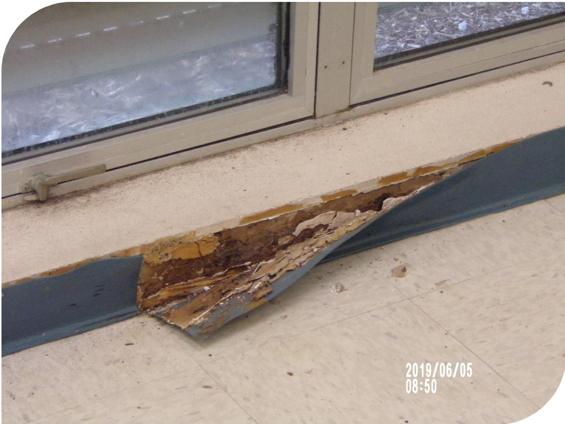
Evidence of termite damage
