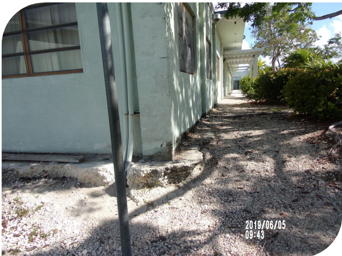
Ground around foundation washed away
