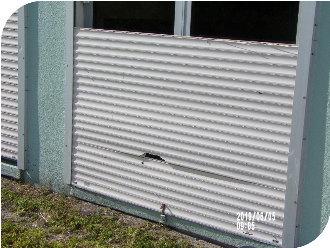
Damage to non-rated storm shutters
