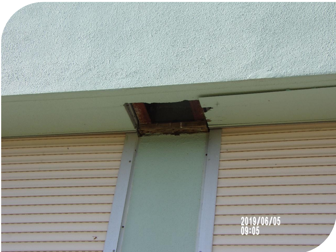
Soffit damage
