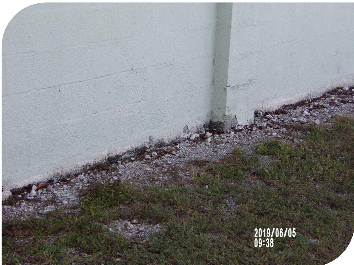
Ground around foundation washed away
