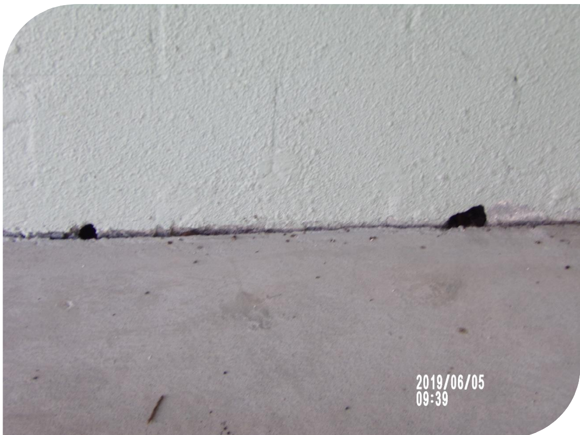
Sidewalk detached from foundation
