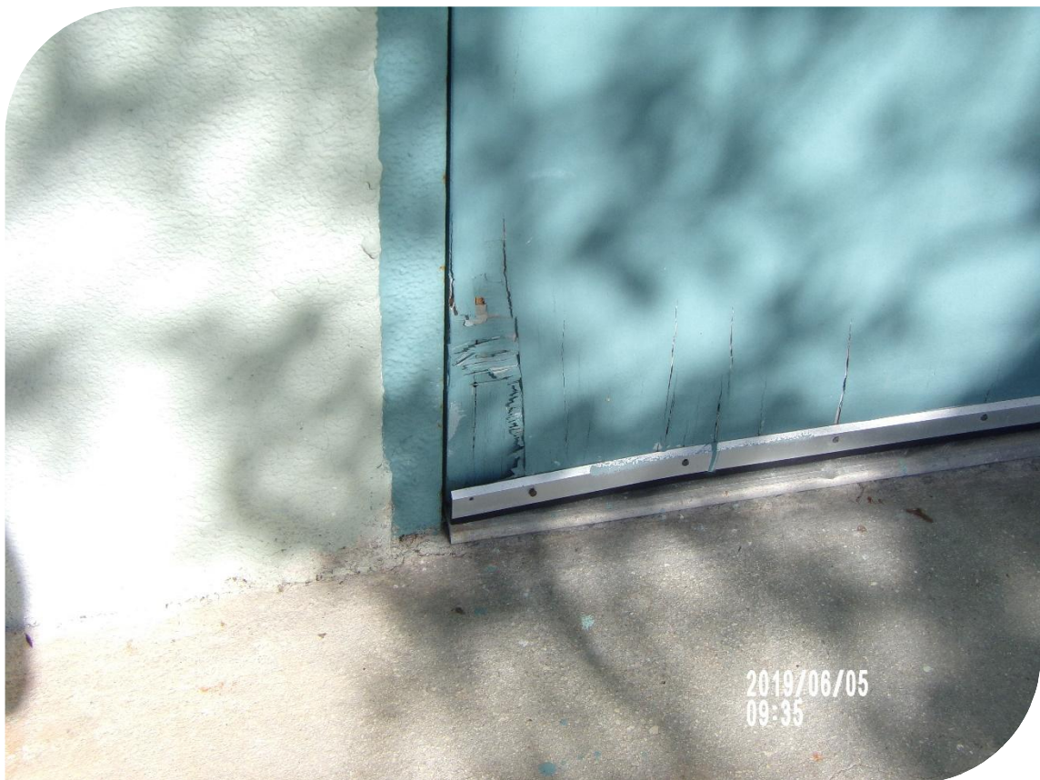
Wood doors with water damage
