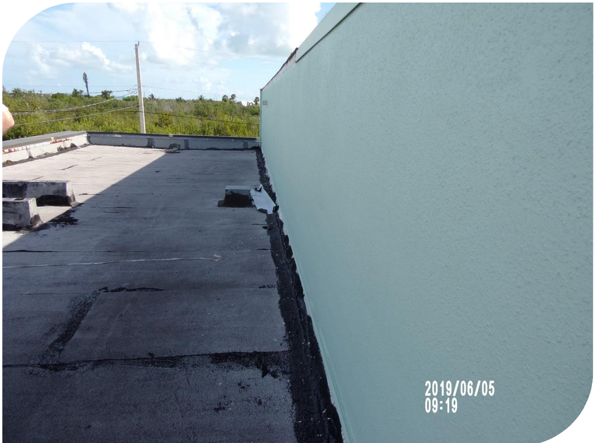
Roof & flashing deteriorated
