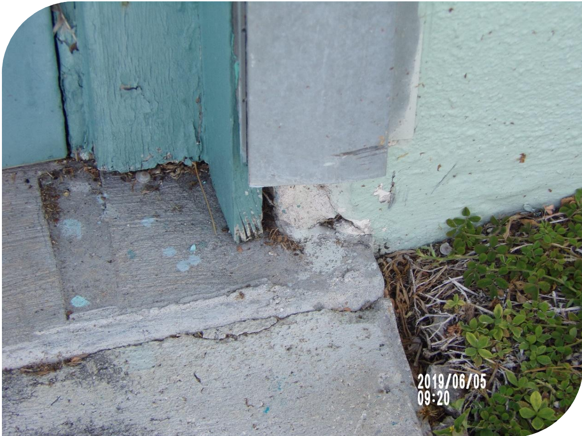
Cracked concrete and degenerating wooden jambs
