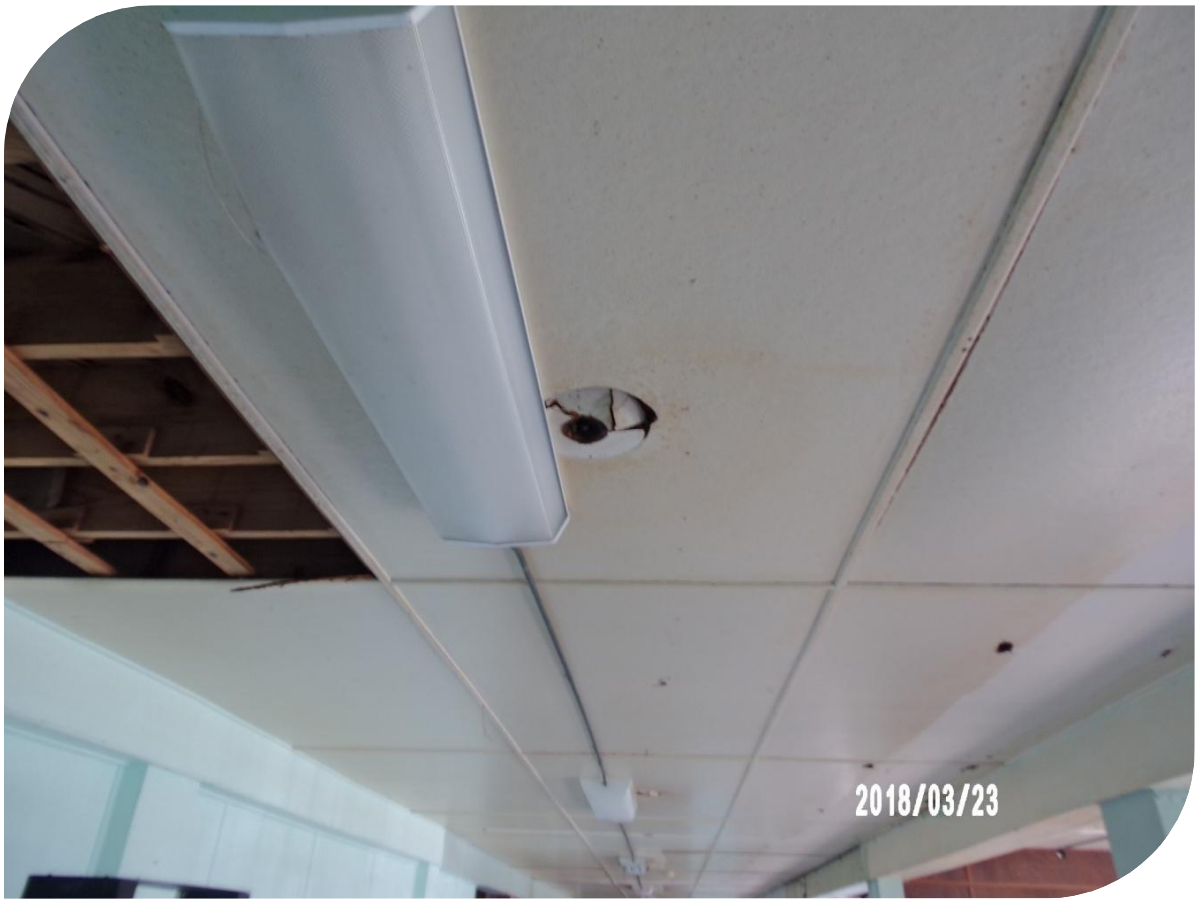
Ceilings missing due to water damage
