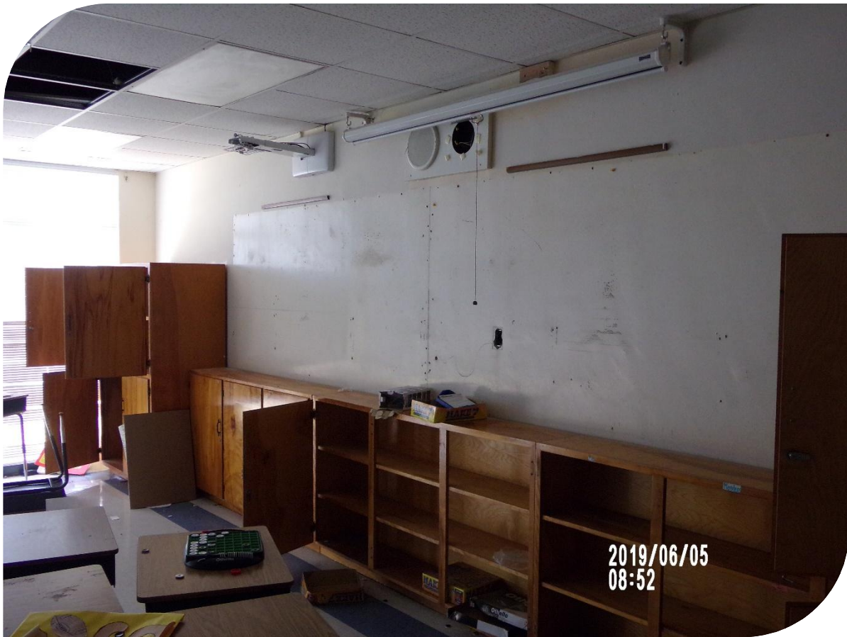
Antiquated casework and moisture intrusion behind white boards
