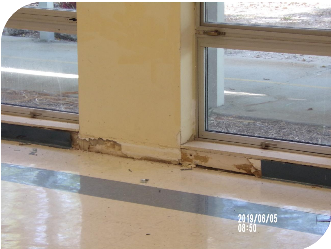
Damage from flooding
