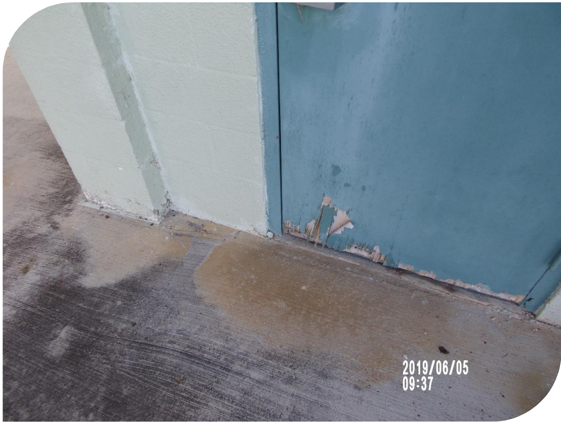
Wood doors with water damage
