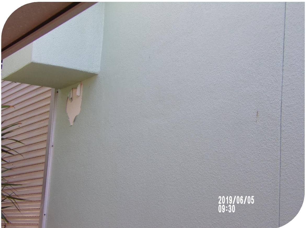
Moisture causing peeling paint
